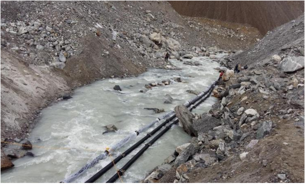
Figure 4: Siphoning of South Lhonak lake, Sikkim (Sharma et al., 2022)
