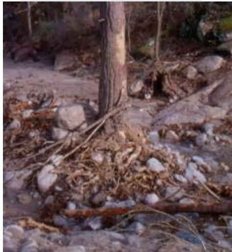
Totally exposed roots
