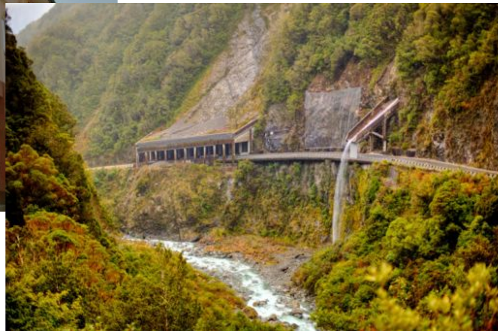
Avalanche and rockfall protection
