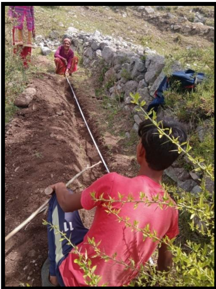
Community members participate in the construction of trenches (recharge pits)
